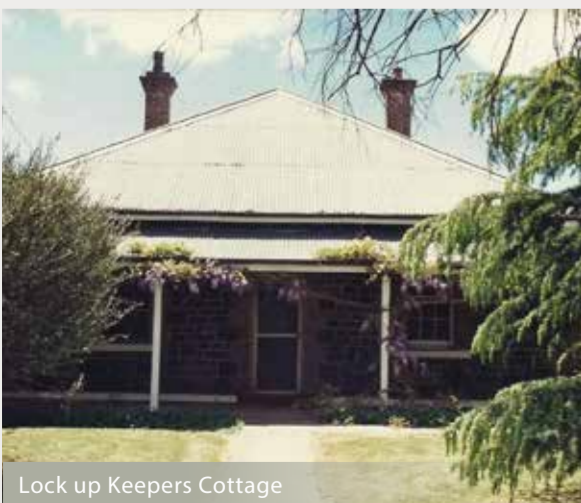
Lock up Keepers Cottage
